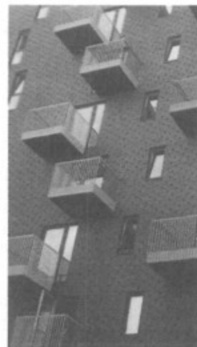
Flats in Barking's Bath House
